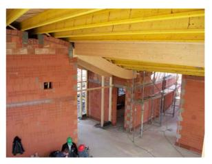
The nursery is an ecological passivehouse. Only building materials that were recommended by the Federal Ministry of Environment were used. At some points we needed to use non-ecological materials and the building owner was willing compromise. The walls, roof and floor have very good insulation (U-Value 0.11).
