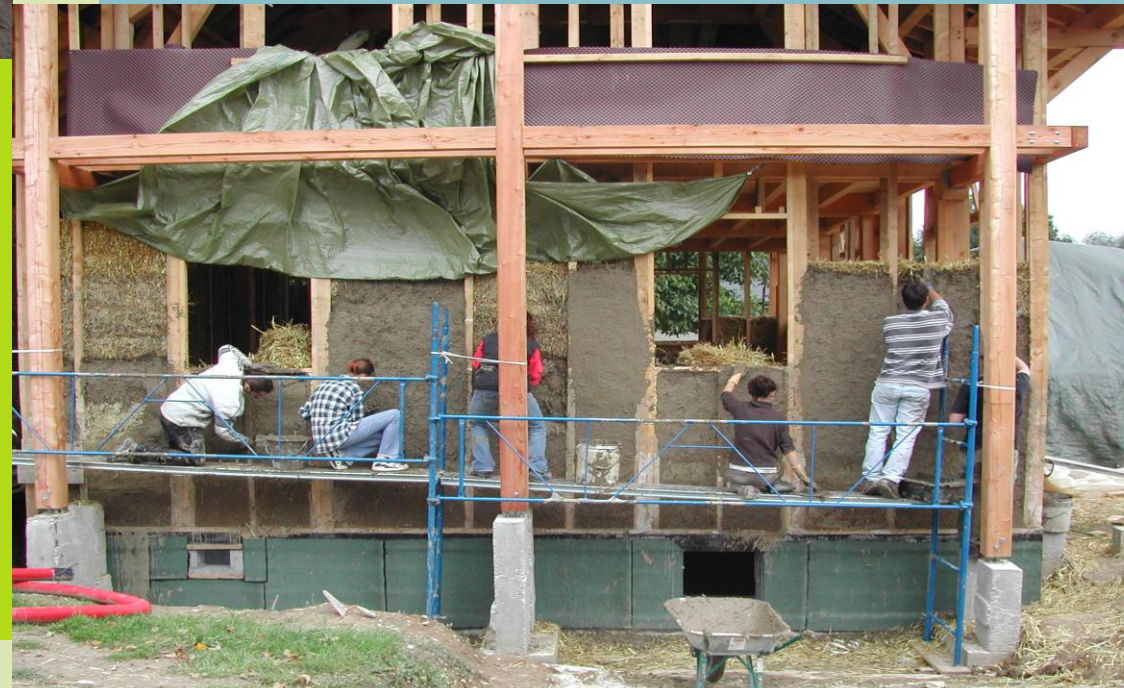
Coating the straw walls
