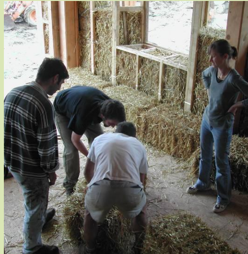
Workshop on straw bales installation
