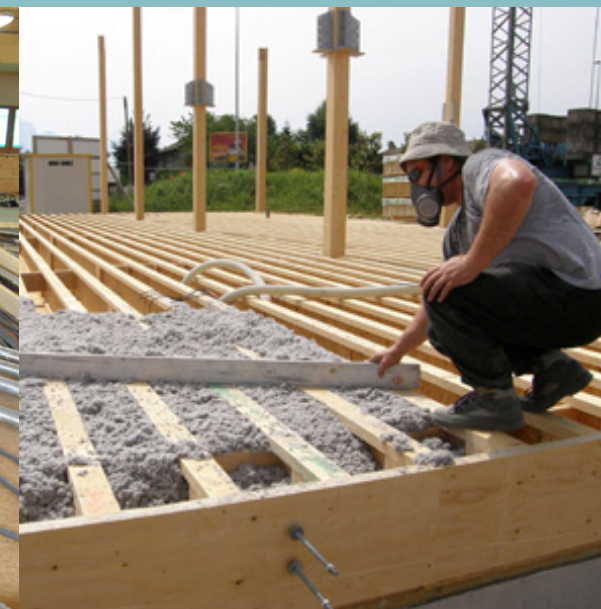
Floor boxes and its insulation (ground floor)
