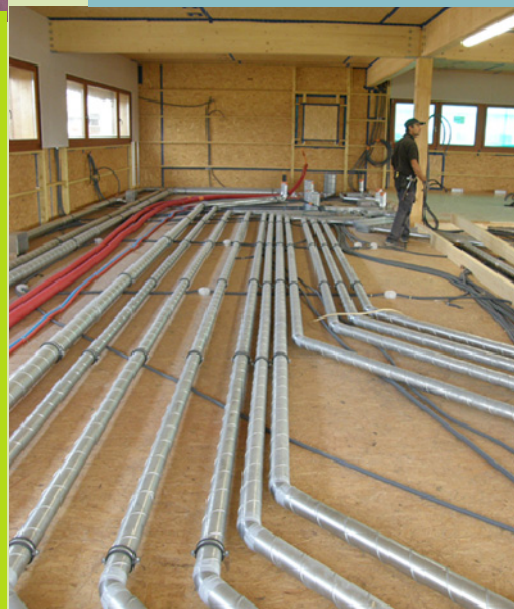
Mechanical heat recovery ventilation
