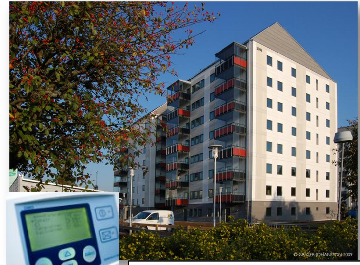
PORTVAKTEN Massive wood frame house in 8 stories with passive house technology
